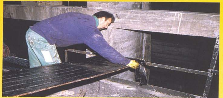
Preparation of SikaWrap ® for flexural strengthening of slab.
