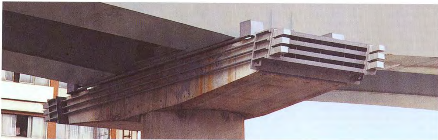
Pier head beam with strengthening by DYWIDAG bar tendons.
