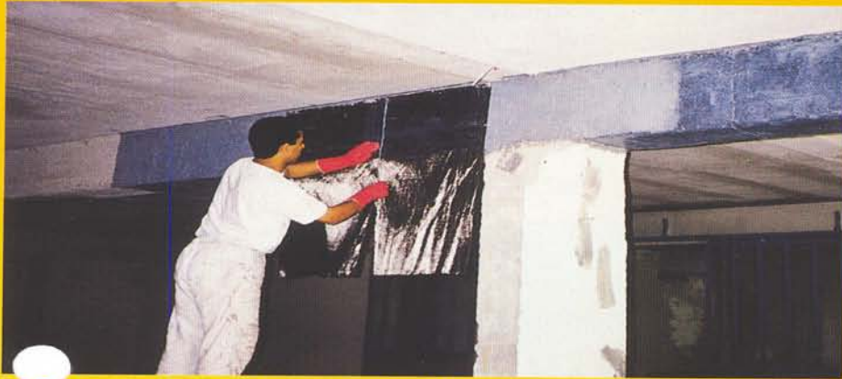
Shear strengthening in a building.
