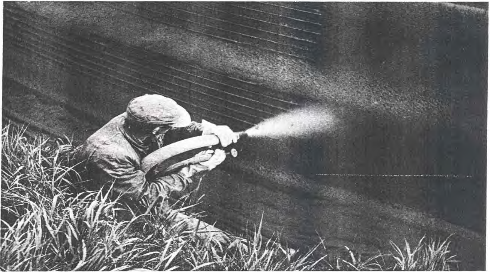
Figure 7.10 Spraying concrete to repair and strengthen settlement tank
