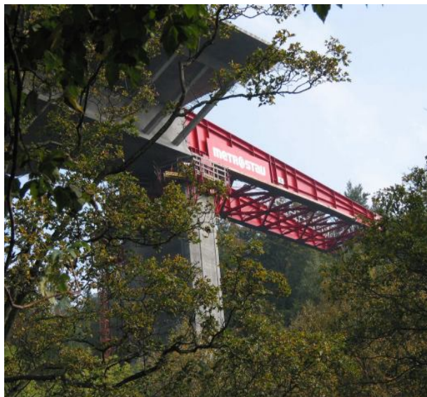
Example of launching nose with I-beams.
