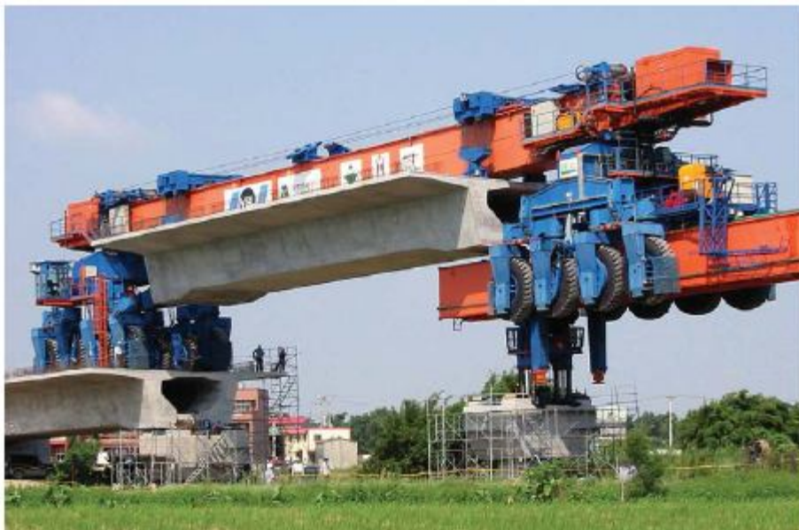
Precast Segmental – Full Span
