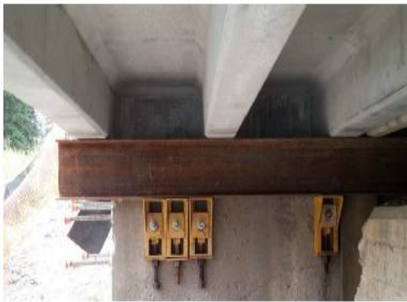
Temporary Widening of Abutment Seat
