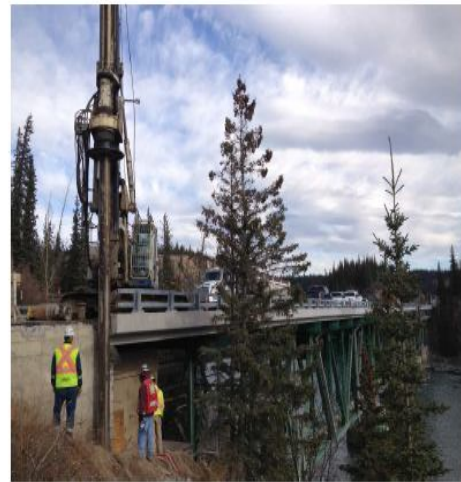
Installation of Abutment Piles
