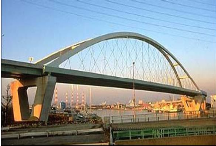
STEEL ARCH BRIDGE
