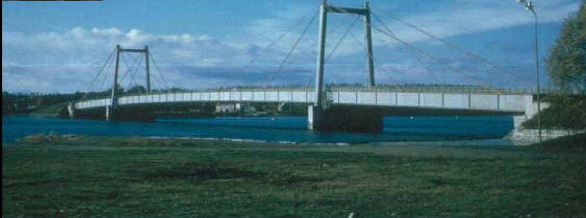
Strömsund Bridge, Sweden
