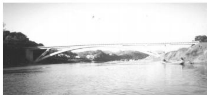
Rigid-frame Arch Bridge
