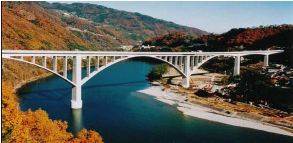
CONCRETE ARCH BRIDGE
