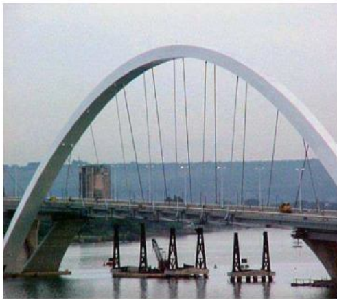
Removal of temporary supports
