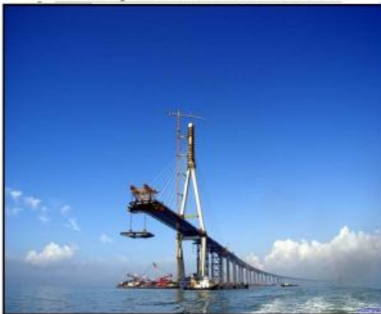
Free Cantilever Method (FCM)
