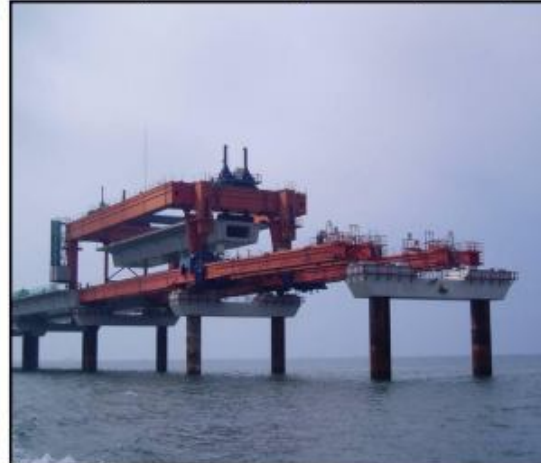
Full Span Launching Method (FSLM)
