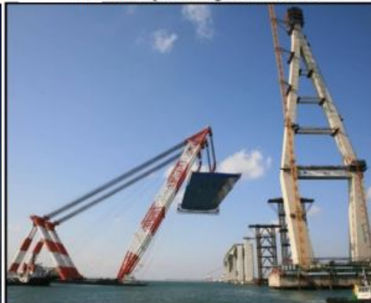
Full Span Launching Method (FSLM)
