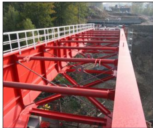
Example of launching nose with I-beams.
