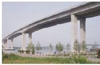
LONG SPAN BRIDGES
