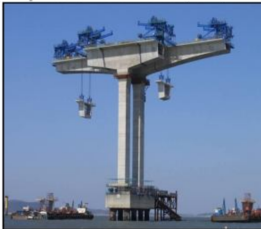
Free Cantilever Method (FCM)
