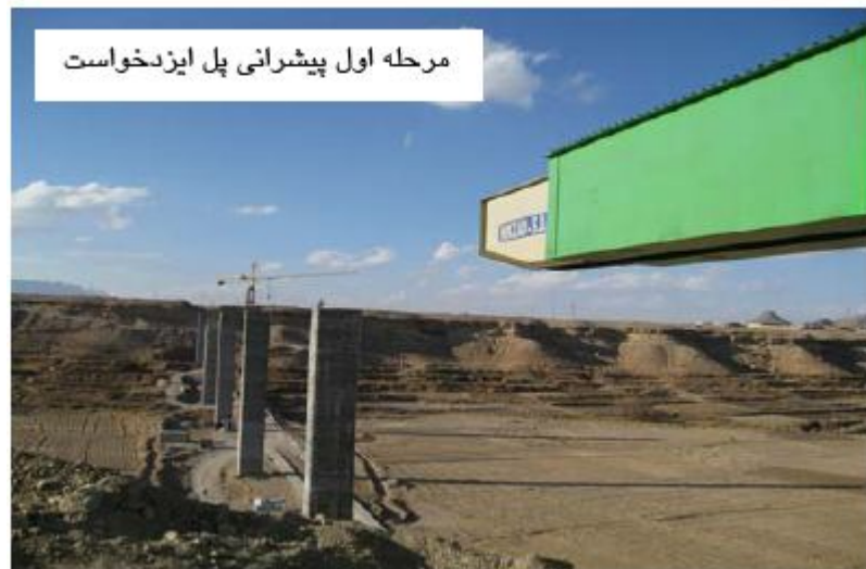
Example of launching nose with I-beams.
