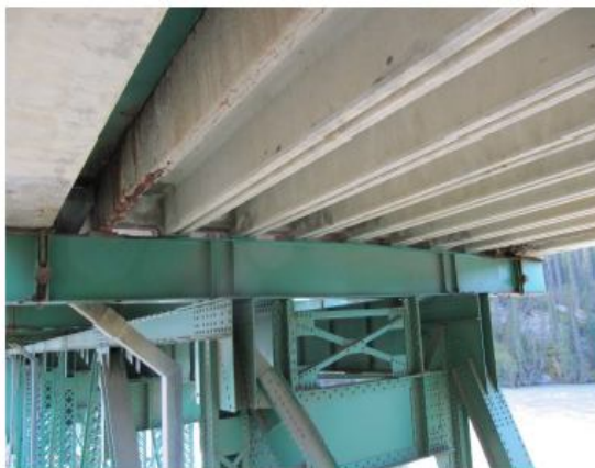
HC Stringers at Truss Expansion Joints
