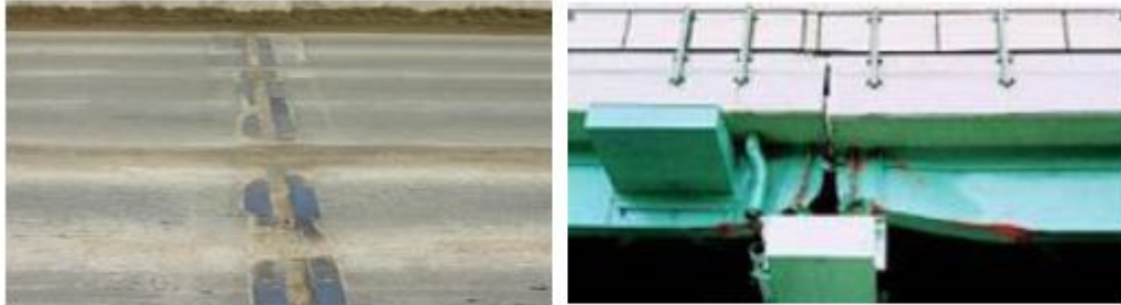
damaged expansion joint bridge
