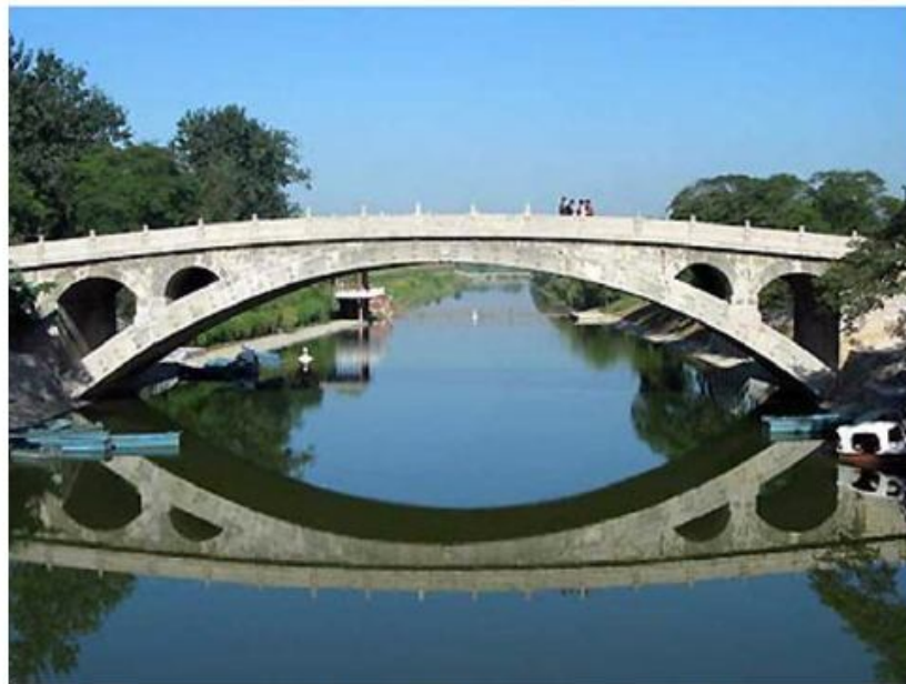
Zhao-Zhou Stone Bridge--A.D. 590-600. Span 37.02 m, rise 7.05m, radius 27.82m, and ring thickness 1.0m,
